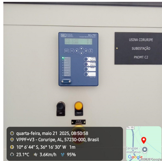
Feeder Protection Relay
